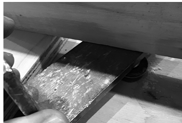
The block can pass through the gap between the anchor pin head and a panel placed on the upper sleepers.
